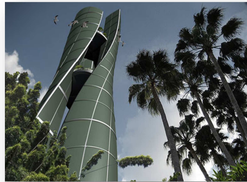
Figure 8. NanoVentSkin on a building.
