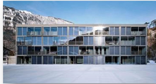
Figure 11. Glass facade (148m 2 ) of Sur Falveng (Leydecker, 2008)
